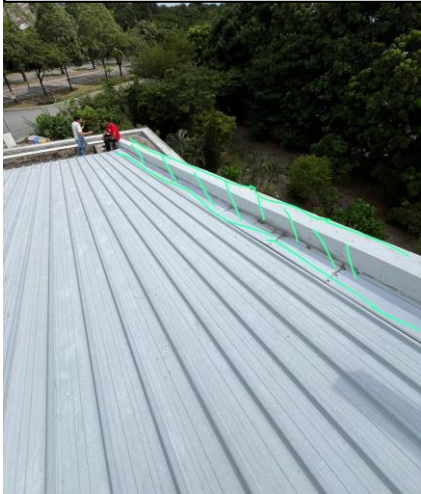
Parapet wall on gable roof.
