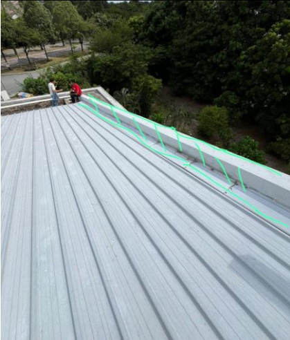
Parapet wall on gable roof.
