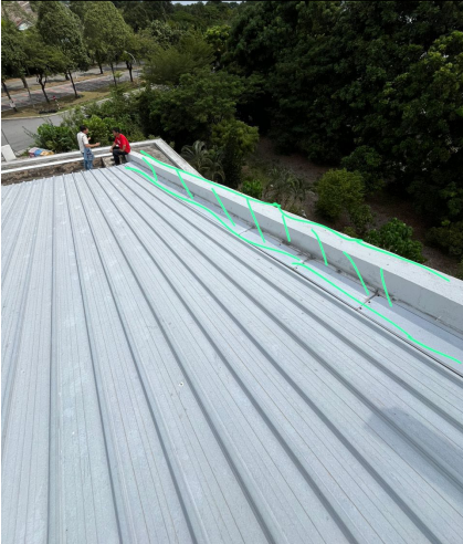
Parapet wall on gable roof.
